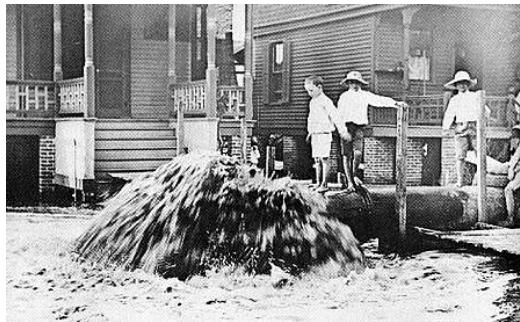
Figure 13. Dredge placement, Galveston.
