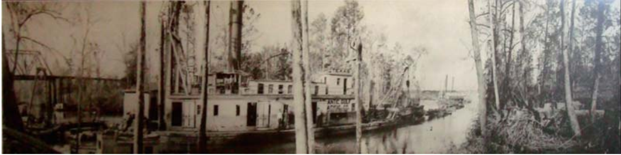
Figure 5. Atlantic, Gulf and Pacific Dredge Texas serving as booster pump for Dredge Pensacola, HSC Turning Basin circa 1928.
