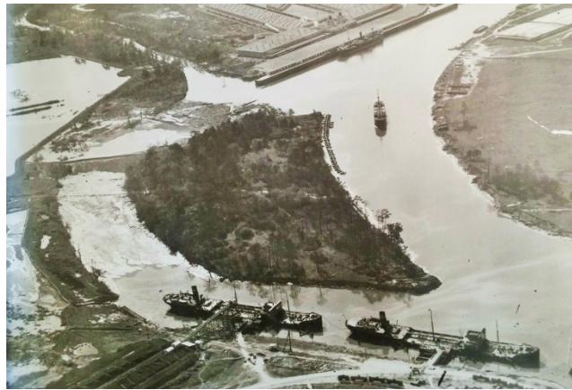
Figure18. Bend Easing after 1913 Dredging.
