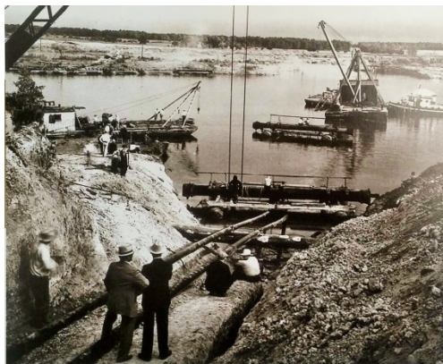
Figure 9. HSC Pipeline Crossing.
