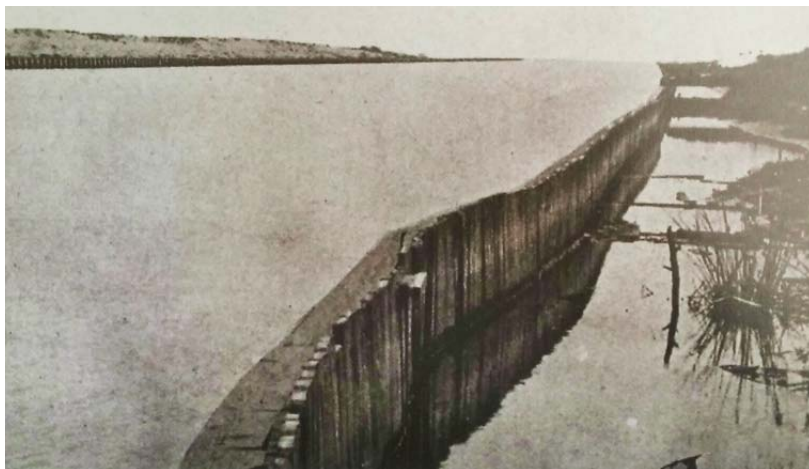
Figure 2. Morgan Cut channel and bulkhead.
