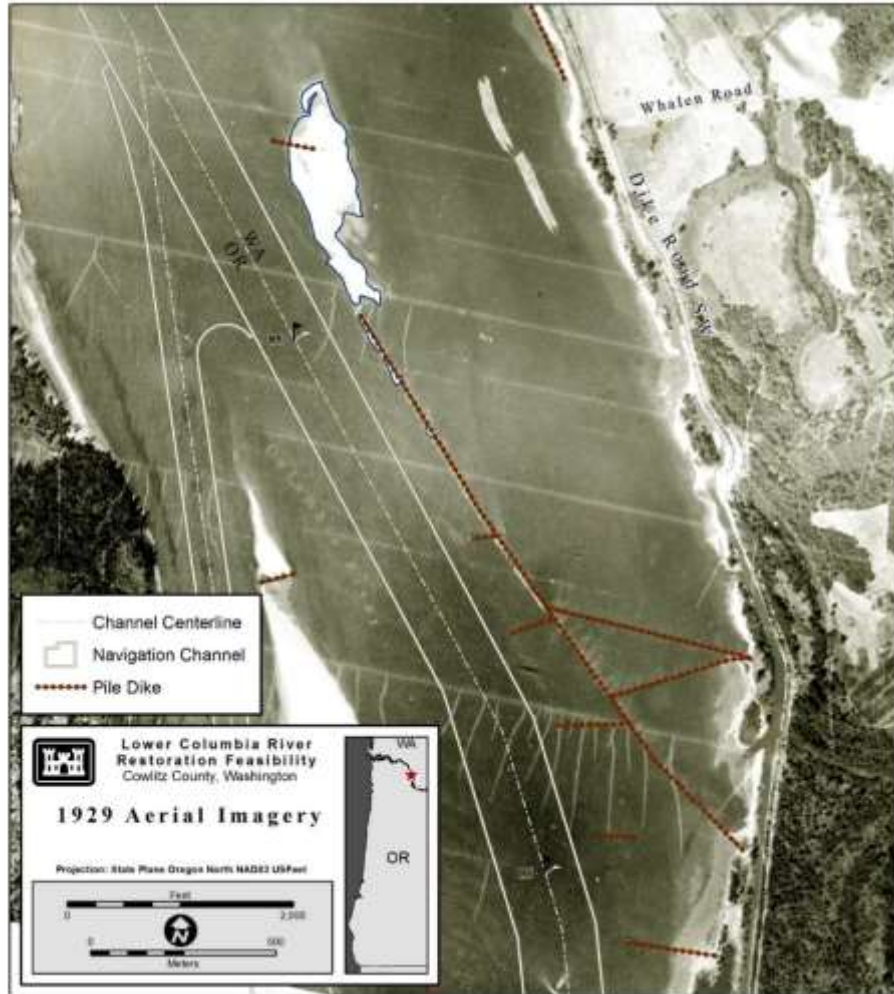
Pile Dike Construction
