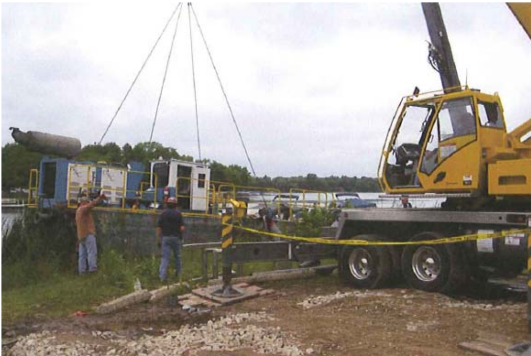
Figure 3. Placement of the 42-foot long DSC 8-inch “Moray” swinging ladder dredge.
