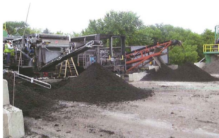
Figure 15. Dewatered sediment off the belt presses.
