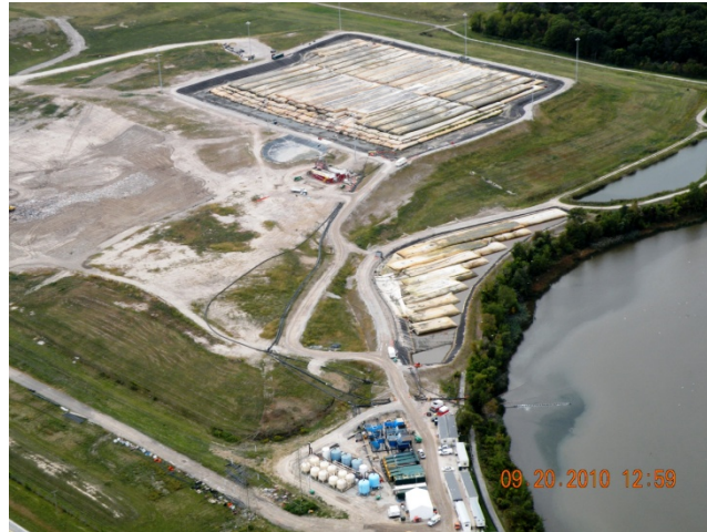
Figure 2. Aerial view of landside operations during active dewatering. The non-TSCA dewatering pad can be seen at the top of the photo, with the TSCA pad below and to the right, and the WTP pad at the bottom of the photo.
