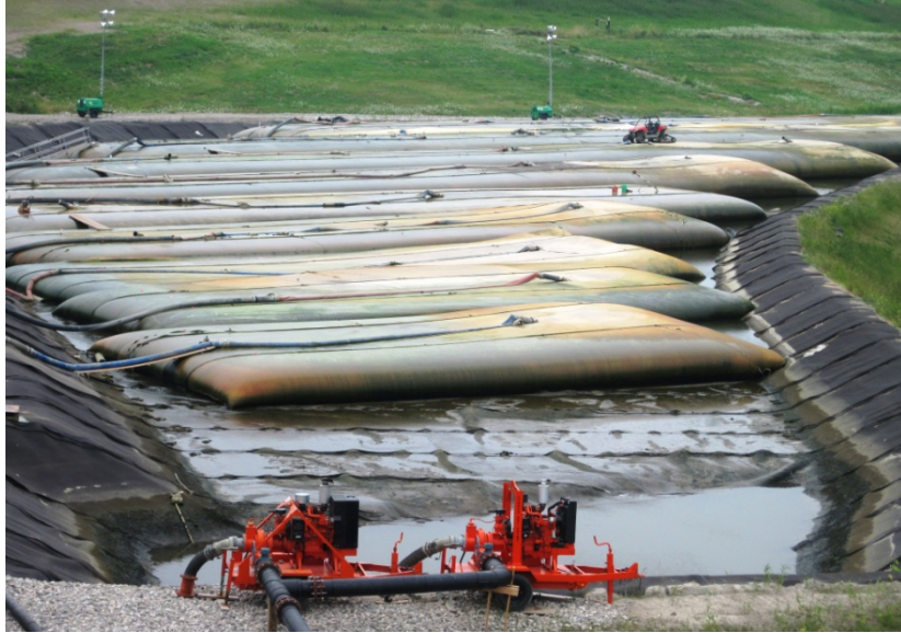
Figure 7. TSCA dewatering pad during active dewatering operations.
