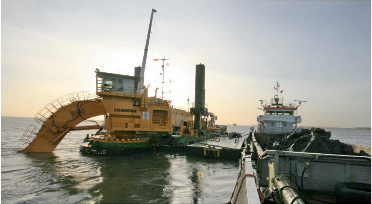
Figure 2. The MP40 pontoon with the Liebherr 995, with one barge alongside.
