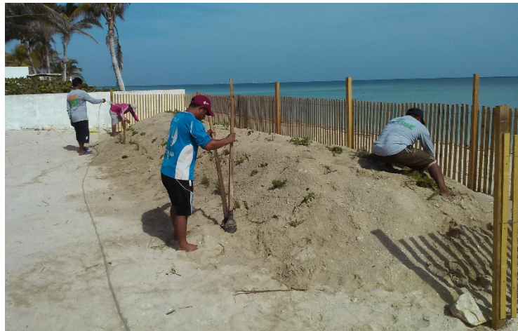
Figure 2. Dune restoration using reclaimed windblown sand, native plant species placement, sand fence installation and application of the PPB SandFirst technology for dune stabilization.
