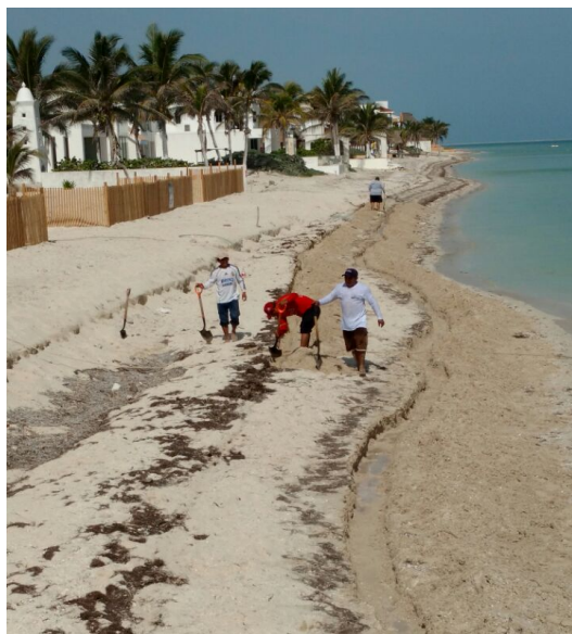
Figure 3. Applying the PPB technology in ditches excavated in the lower part of the beach (berm).
