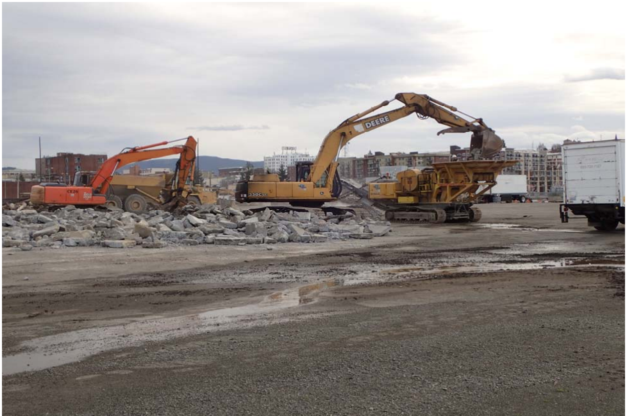
Photograph 3. Concrete Crushing and Upland Stockpile for Material Reuse
