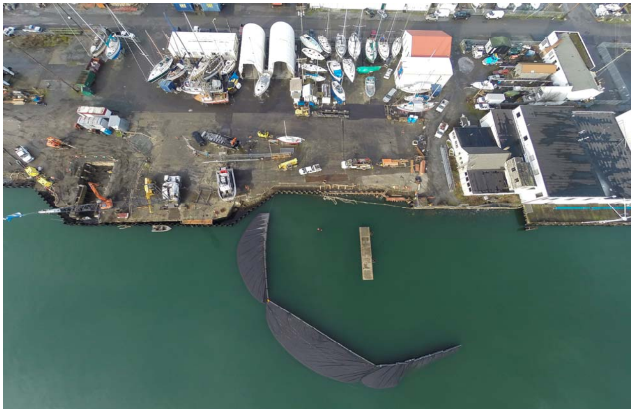
Photograph 1. Silt Curtains for Water Quality Control
