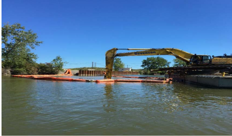
Figure 9. Shallow-water dredging with double turbidity curtains deployed, without the moon pool.
