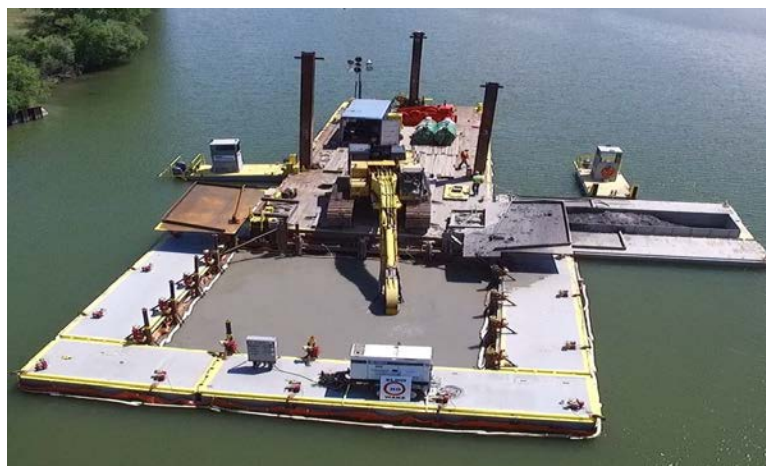
Figure 7. Derrick barge with attached moon pool and drip pans in use.
