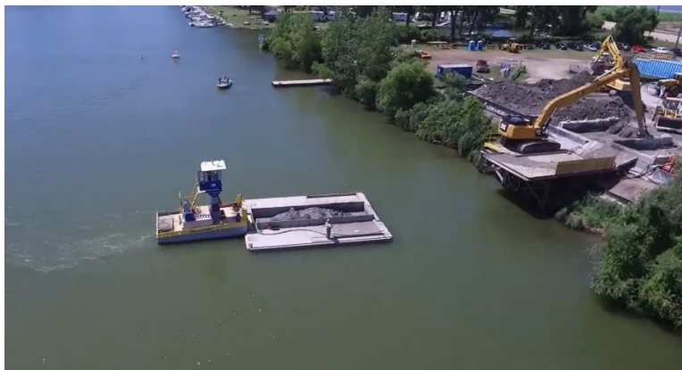
Figure 10. Transporting a full barge of sediment from the NAPL Area to the SPA and offloading area.
