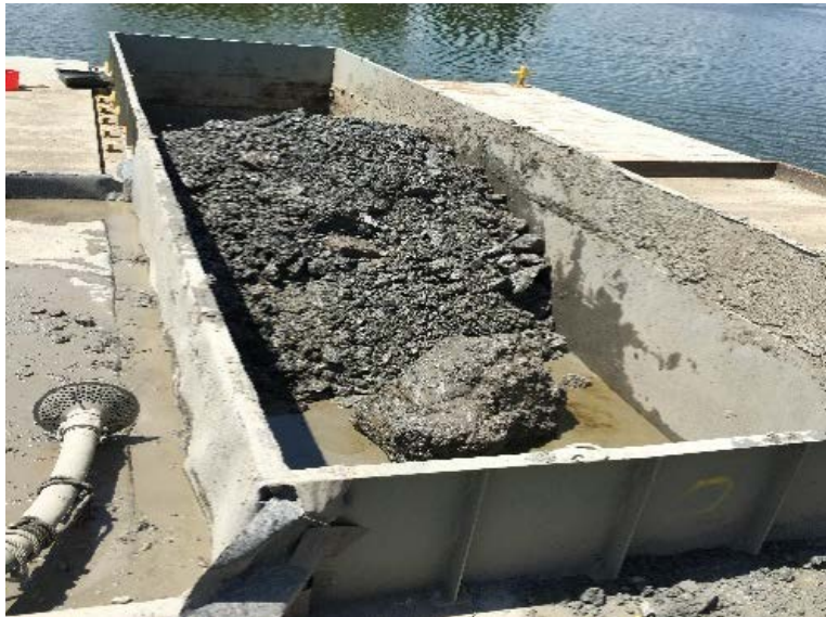
Figure 5. Barge of hard friable rock typically found at greater dredge depths.
