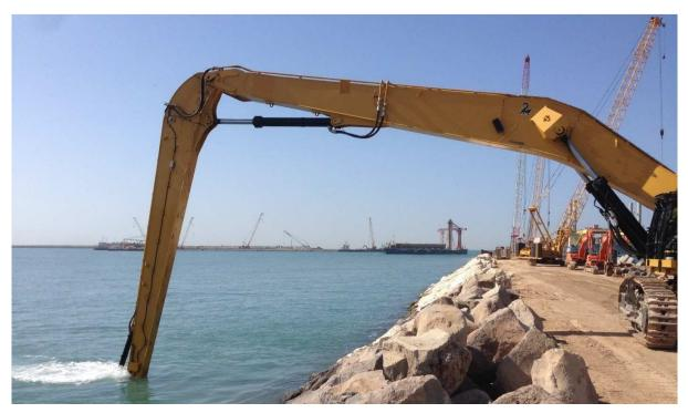
Figure 5. Customized 29 m (95 ft.) long-reach excavator at work in breakwater construction.
