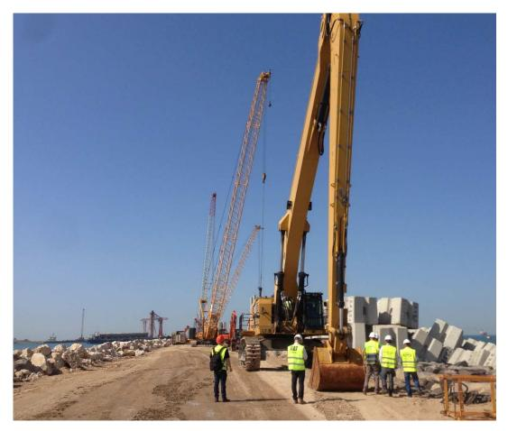
Figure 4. Customized 29 m (95 ft.) long-reach excavator at breakwater site.
