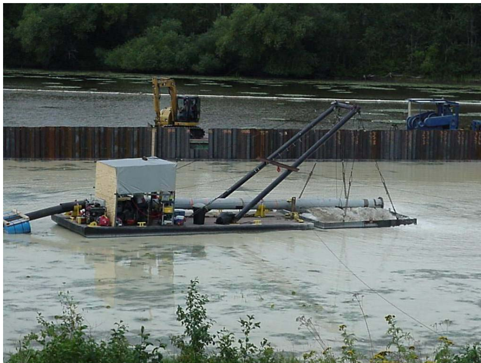
Figure 1. Sub-capping operations.
