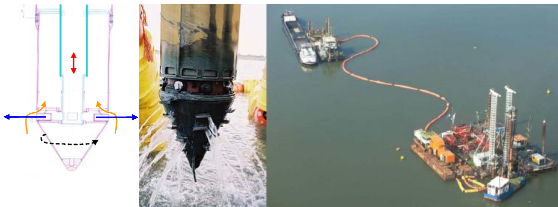
Figure 3. SSD “Sub-o-Suction” (Ballast-VanOord): Outline, drill head and offshore plant
