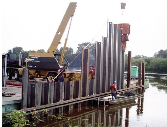
**Figure 4. Environ designed and installed a sheet pile wall, which was constructed to contain a surcharge sand cap designed by the SERVICE.**
