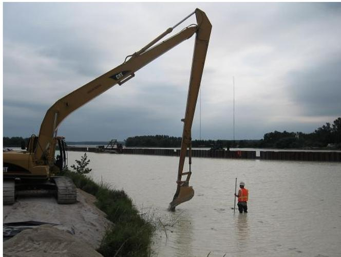
**Figure 6. An alternative shoreline cap placement method, approved by the CQA/environmental monitoring engineer, included placement of uniform lifts by the RAC using a long-stick excavator.**
