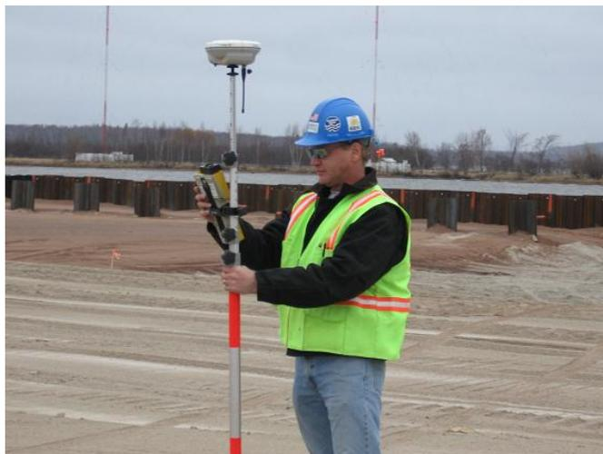
**Figure 8. The CQA/environmental monitoring engineer surveyed each cap lift thickness to ensure compliance with project specifications.**
