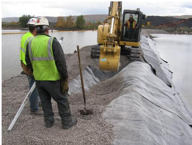
**Figure 3. An alternative geotextile clay liner (GCL) tie-in and CAD end dike top completion was successfully approved through cooperative project management channels.**
