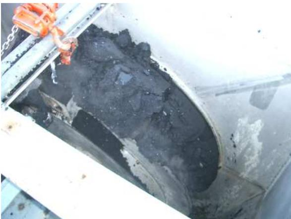
**Photograph 10. Discharging dewatered sediment through outlet.**
