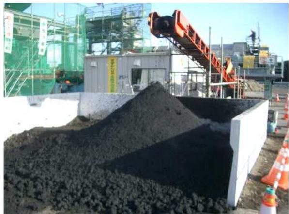
**Photograph 11. Discharging dewatered sediment to a pit.**
