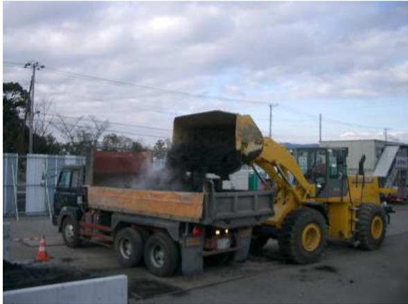
**Photograph 12. Loading dewatered sediment.**
