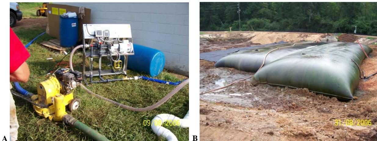
**Figure 12. A) Injection of polymer with a WaterSolve WSLP-4800USF make-down unit. B) Due to limited processing space, the south storage lagoon was used for the Geotube® lay-down area after initial excavation of biosolids into the north lagoon.**
