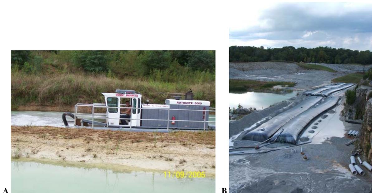
**Figure 8. A) Retention basin sediments were dredged by Kentucky Dredge's 8-in Crisafulli Rotomite 6000 auger dredge. B) Solve 9350 was used to contain, dewater, and consolidate 850 gpm aggregate sediments in 45-ft circumference Geotubes®.**
