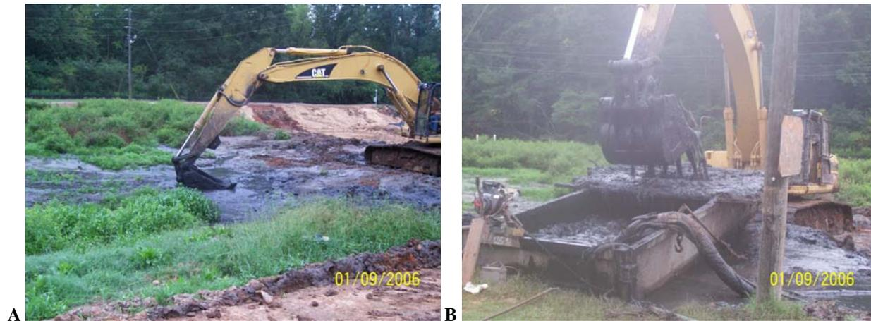
**Figure 11. A) Mechanical excavation of vegetation and other debris from a 1-MG biosolids storage lagoon prior to hydraulic dredging of sludge (B) to Geotubes® for further processing (i.e., dewatering and consolidation).**
