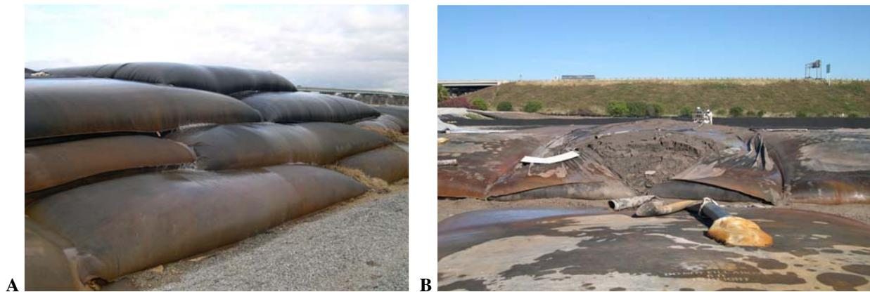
**Figure 6. A) Four layers of 60-ft circumference Geotubes® of decreasing length were used to maximize processing and storage capacity. B) Sampling and excavation of PCB-contaminated sediments for disposal at a licensed local landfill.**
