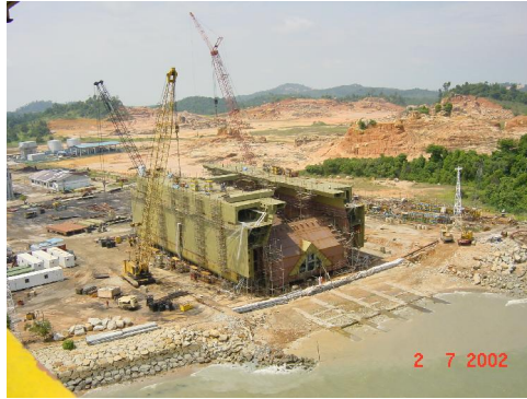
Fig. 33 Section in progress
