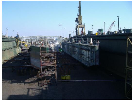
Fig. 27 pontoon separated into two parts
