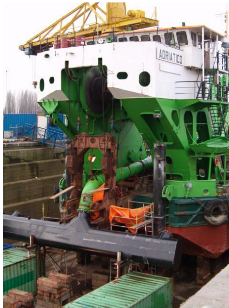
Fig. 13 T-shaped pipe on the ladder
