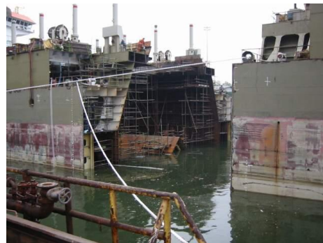
Fig. 34 separation in dry dock
