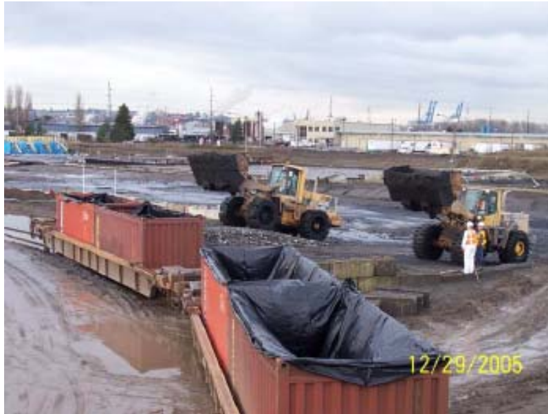
Figure 7. Lined railcars staged for loading from the sediment stockpile area (Photo Courtesy of DOF, Inc.).
