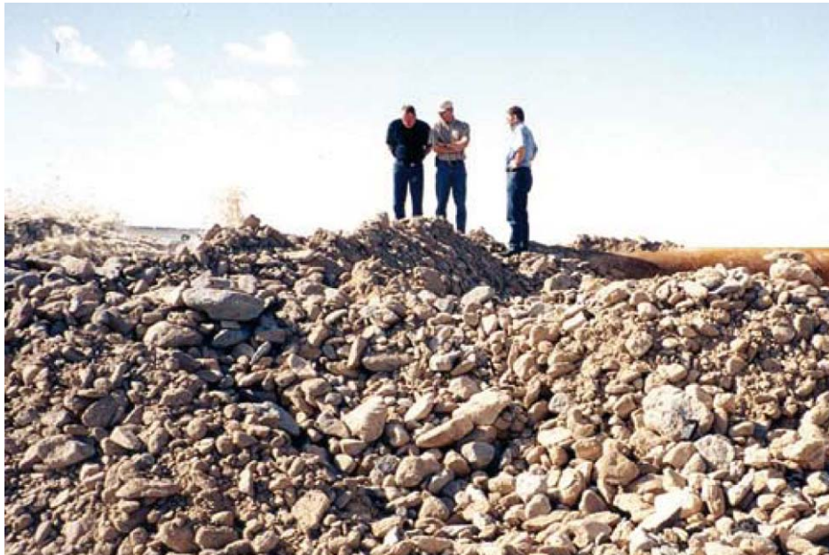
Figure 6. Shore deposit filled with large sized material by a heavy duty cutter suction dredger.
