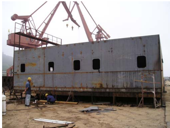
Figure 8. Accommodation deckhouse under construction.
