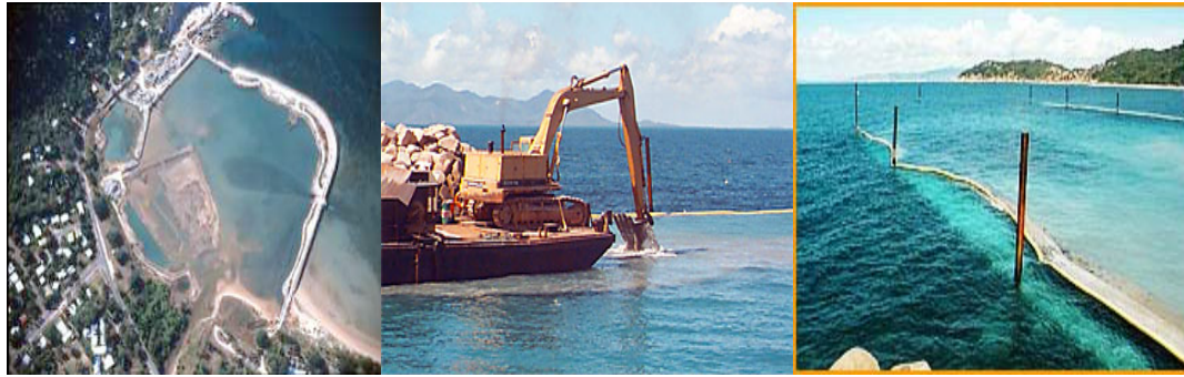
Figure 3. Dredging a navigation channel to a marina using barge-mounted grab and silt curtains to minimise impacts to adjacent coral.
