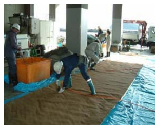
Coconut mat attached using hook rings
