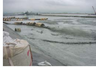
Condition after filling with dredged soil
