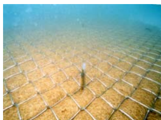
Installation of AMAMO sheet completed
