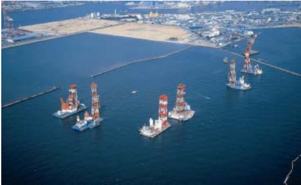
Figure 10. Soil improvement work with six work vessels.
