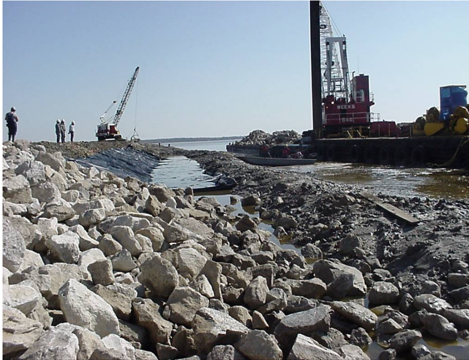
Figure 4. Rock shore protection with geo-membrane.
