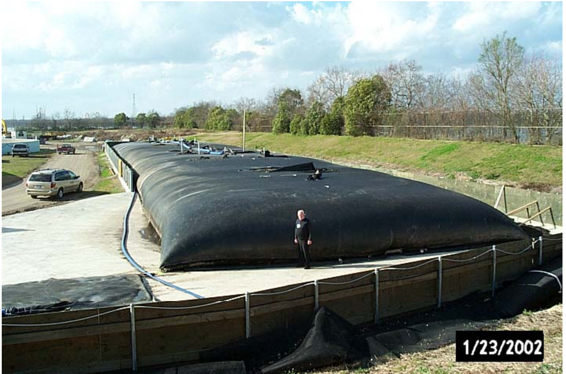
Sewage Sludge Filled Tube
