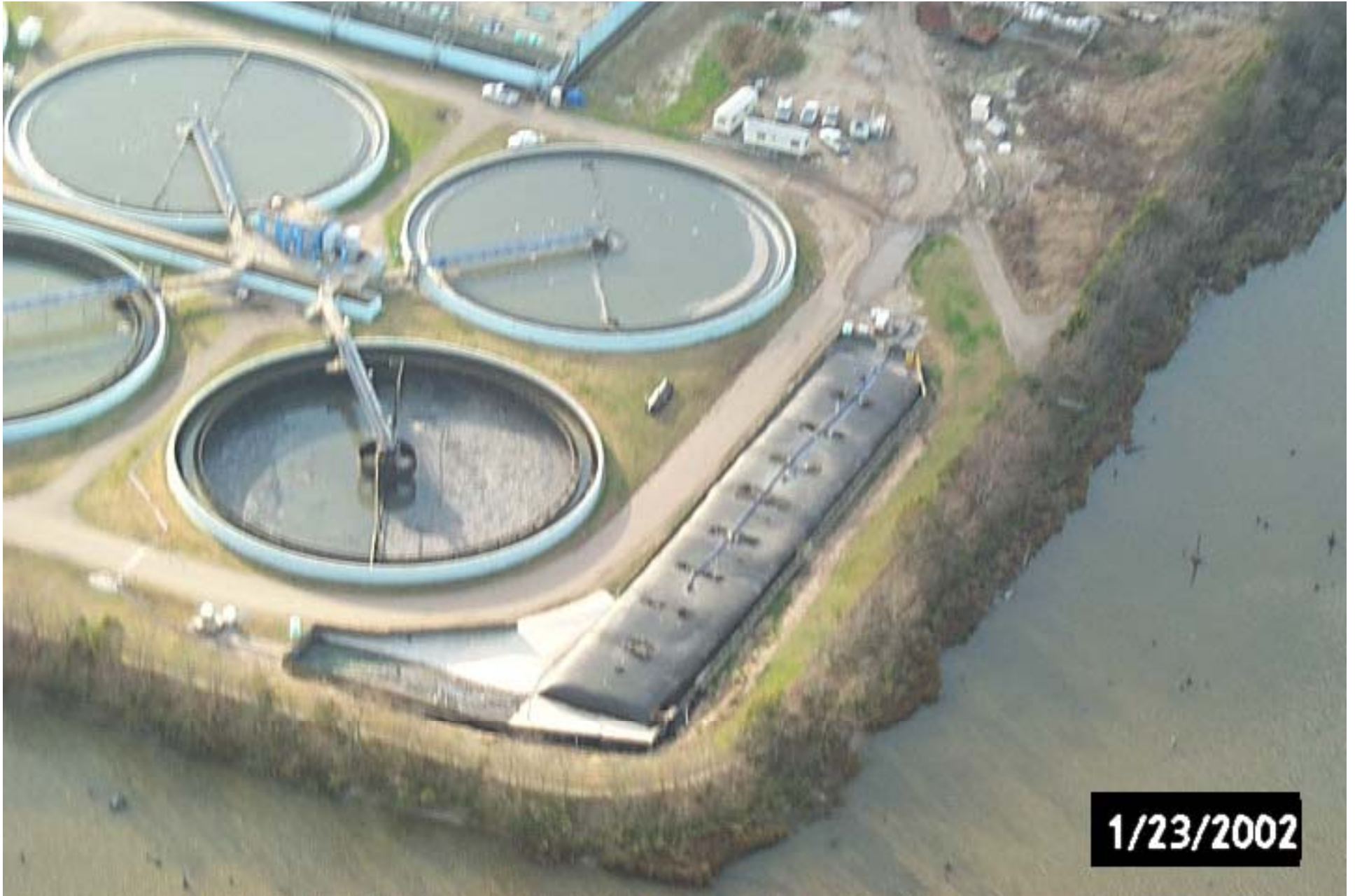
Aerial View of Sludge Filled Tube
