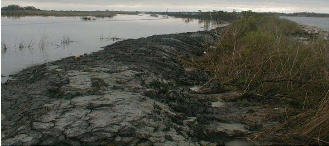
Figure 9. Sacrificial Earthen Guide Dike – Area “B”.
