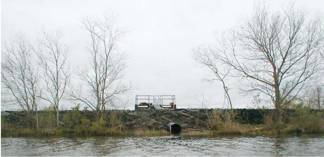
Figure 11. CDF Area SB-S –CDF Dike and Weir Structure.
