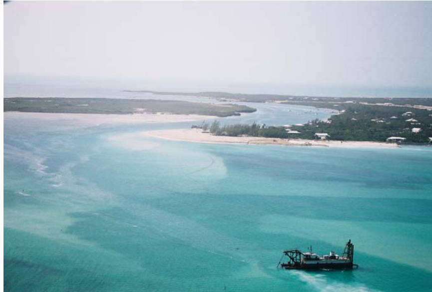
Figure 3. Dredge in operation with Beach fill and Leeward-going-through in background
