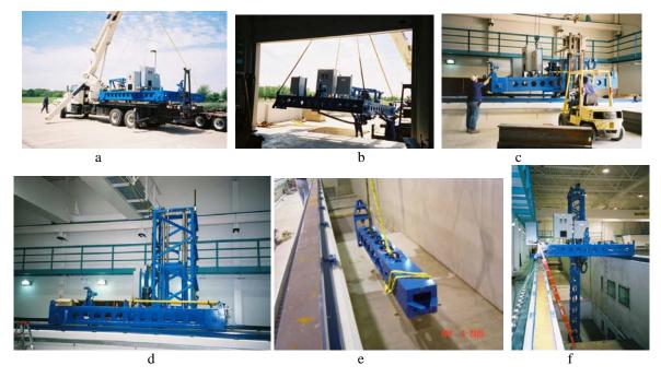
Figure 10. Dredge/tow carriage installation sequence.
