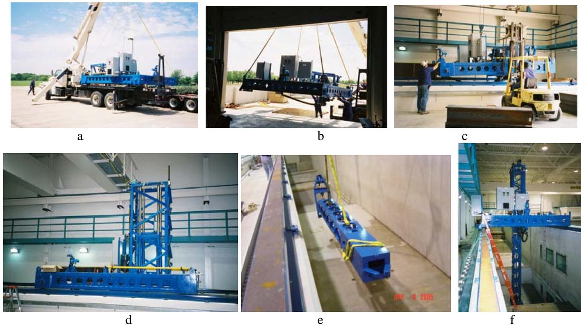
**Figure 10. Dredge/tow carriage installation sequence.**
