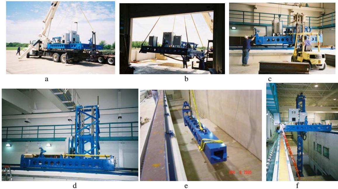
**Figure 10. Dredge/tow carriage installation sequence.**
