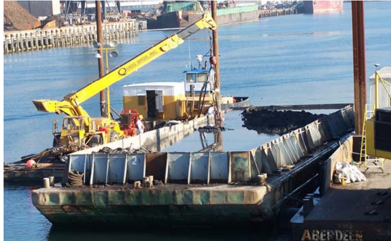
Figure 2. Barge dewatering system.
