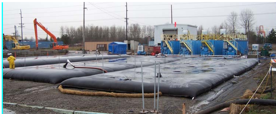
Figure 4. Geotubes with mixing tanks in background.
