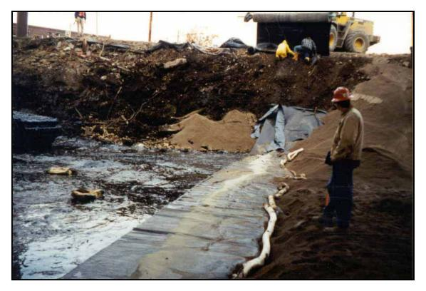
Figure 6. Placement of the geosynthetic clay liner.
