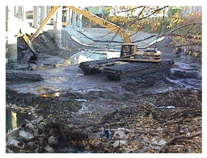
Figure 5. Photograph of amphibious excavator removing impacted sediment.
