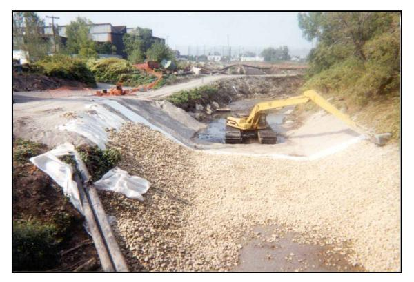
Figure 7. Placement of sand and stone cap elements.
