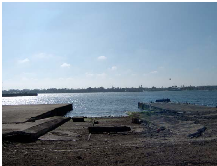
Figure 4. Abandoned shipways area, showing mole pier (left) and marine railway (center).
