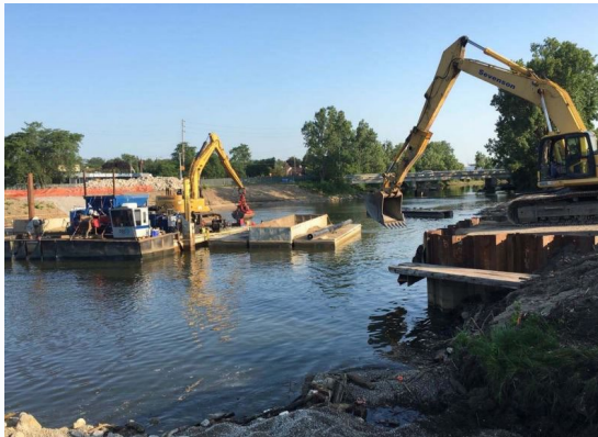
Blended Barrier for River MGP Sediment Remediation
