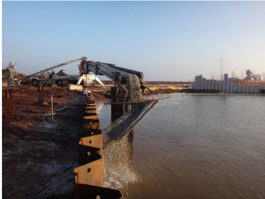
Sealing Bulkhead Wall to Limit Upland Residual Contaminant Migration
