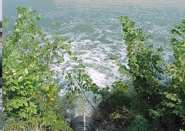
Figure 17. Geotube® weep being returned back to the waterway
