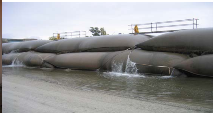
Figure 21. Geotubes filled with flocculated solids and draining
