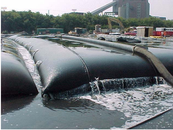
Figure 16. Geotubes being filled with flocculated solids and draining
