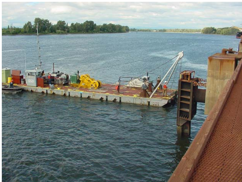
Figure 6. Terminal 5 Berth 503 underwater grading.
