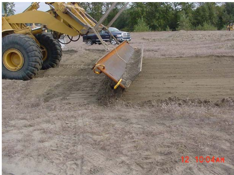
Figure 9. Upland grading test.
