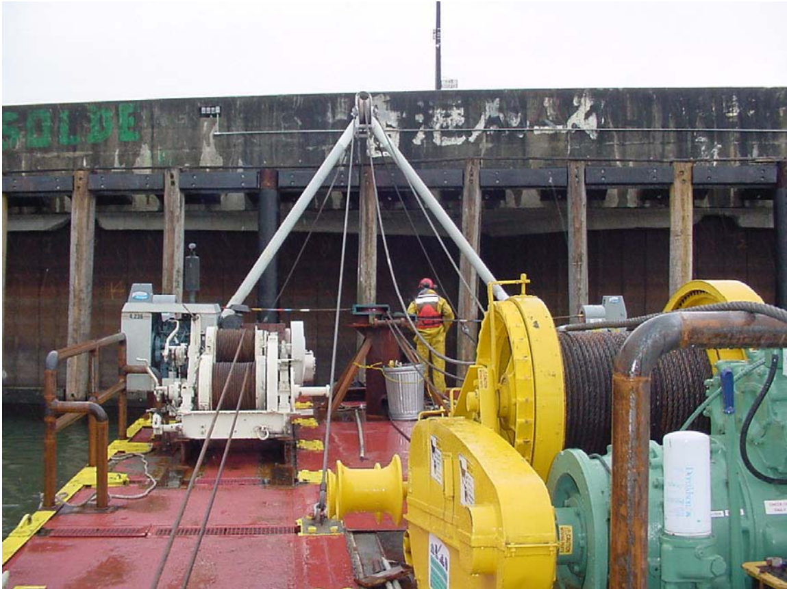
Figure 4. Lifting and positioning winches.
