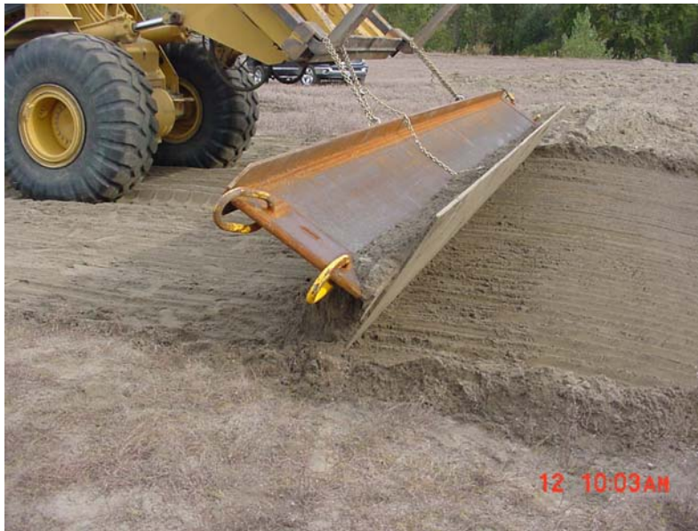
Figure 8. Upland grading test.
