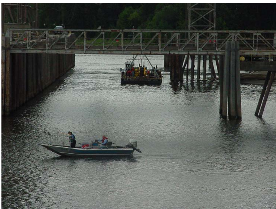
Figure 10. Water quality monitoring (foreground) during grading operations (background).
