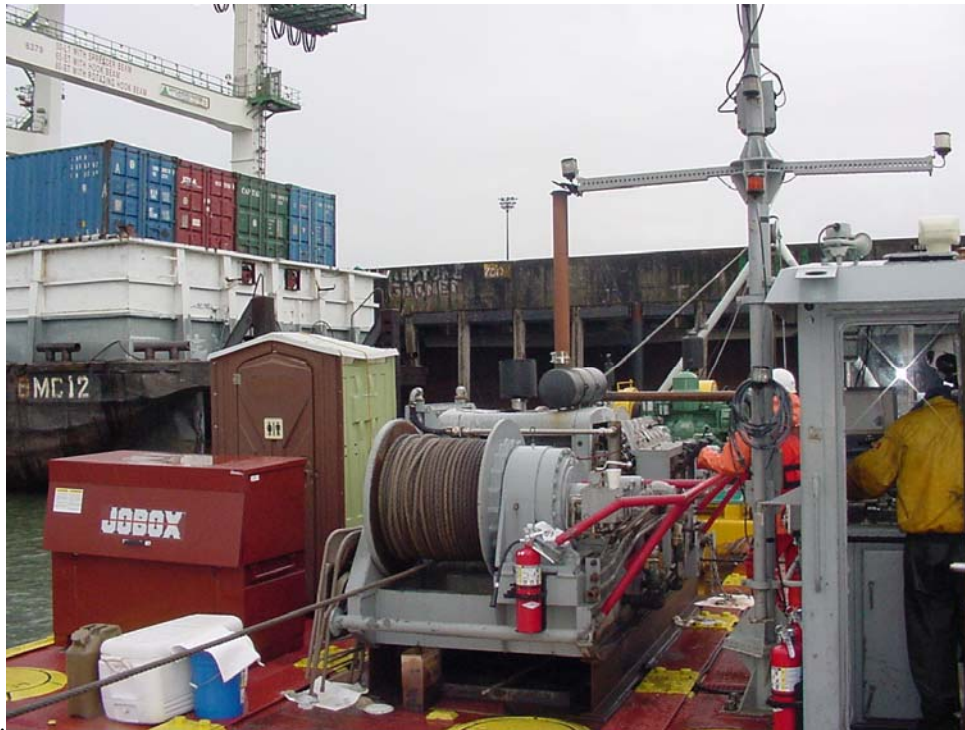
Figure 7. Terminal 6 grading operations.
