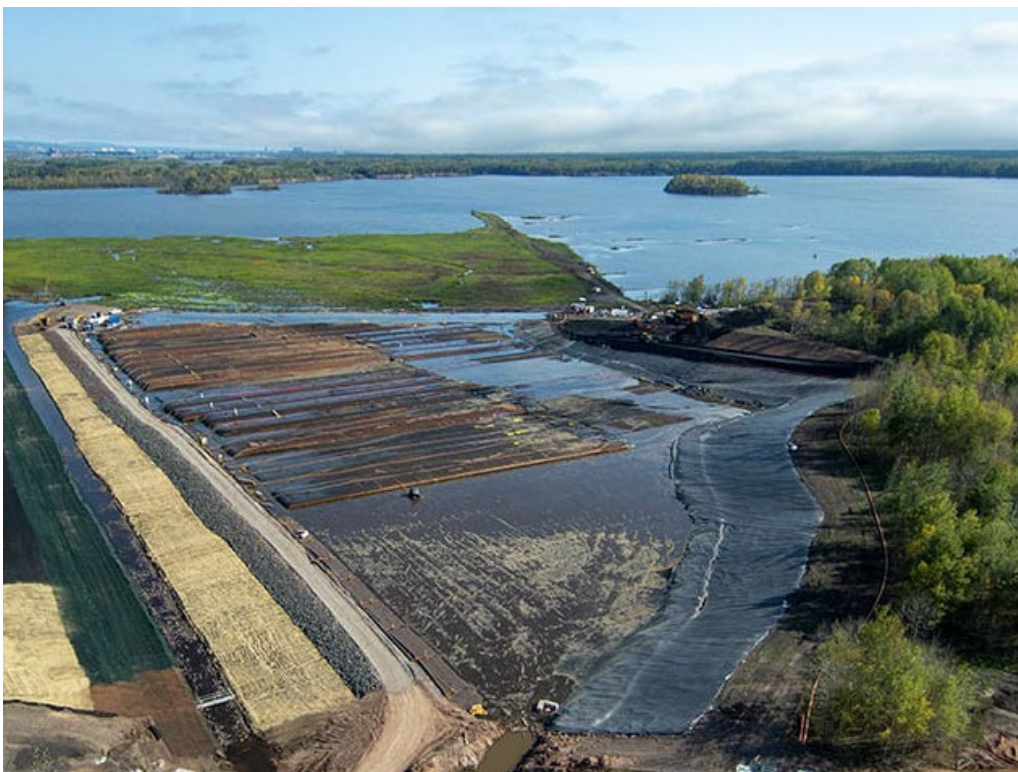
Upland CDF with Geotube® bag field in progress (2021)
