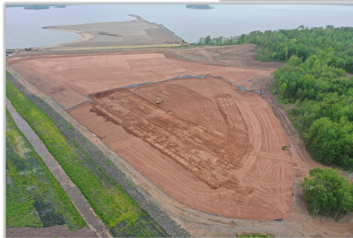
Upland CDF with final cap being placed (2023)
