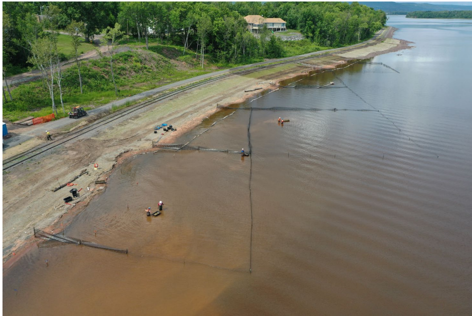
Planting in shallow sheltered bay with predation exclusion fencing
