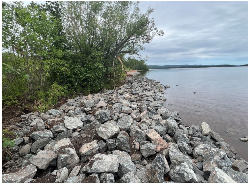
Critical shoreline protection in areas prone to high erosion
