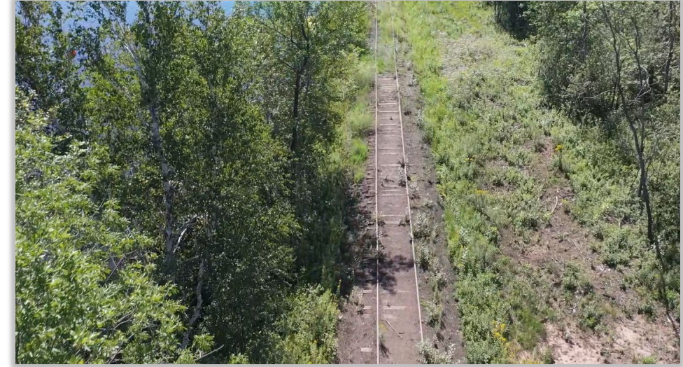
View of a section of the LSMRR pre-project construction
