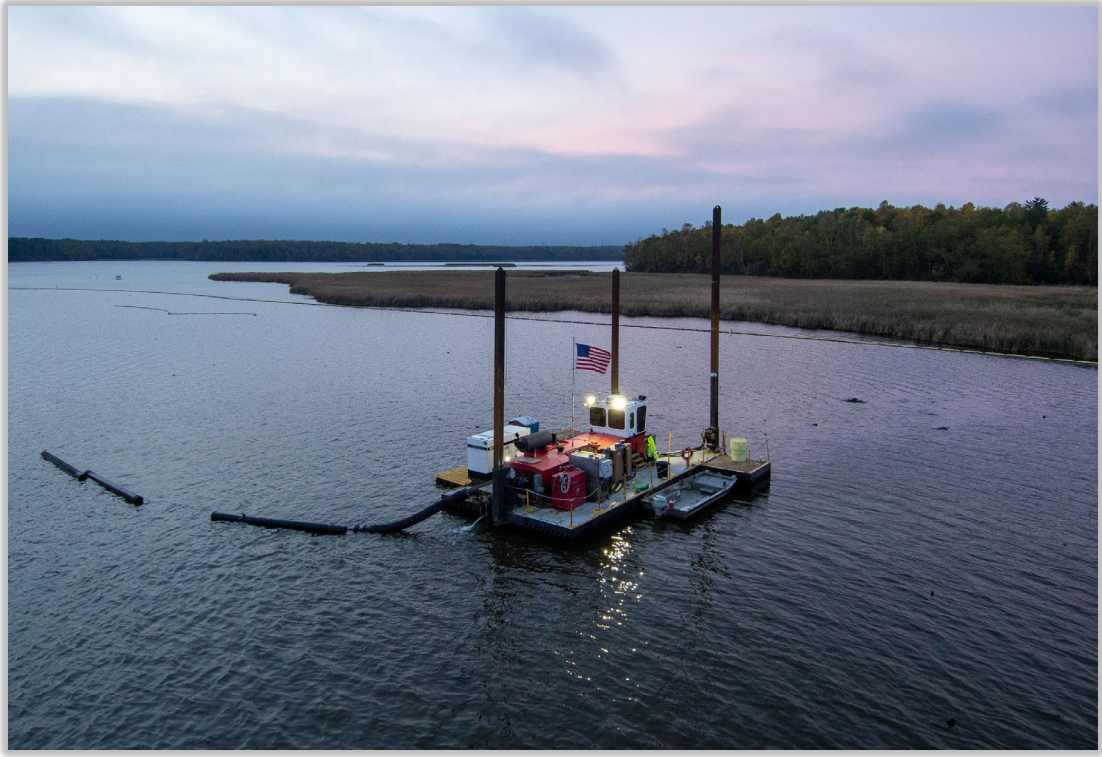
Hydraulic dredging in Wire Mill Delta
