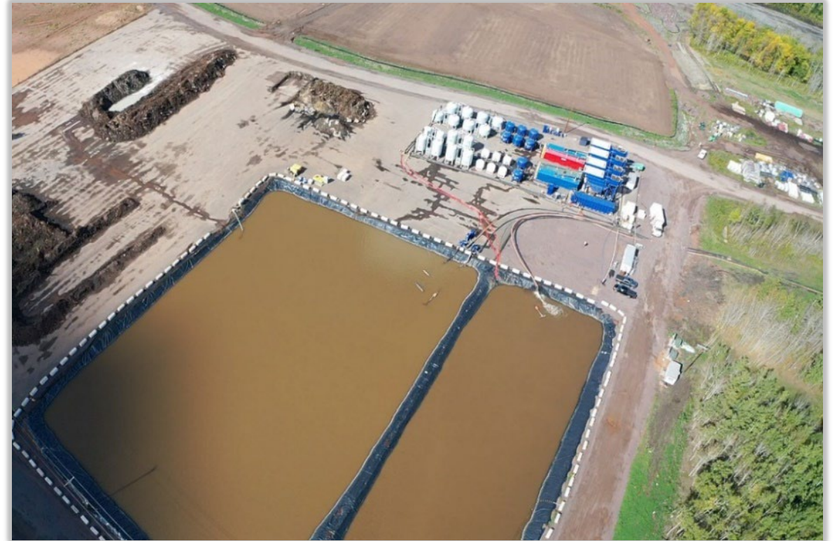
Aerial of the onsite water treatment plant
