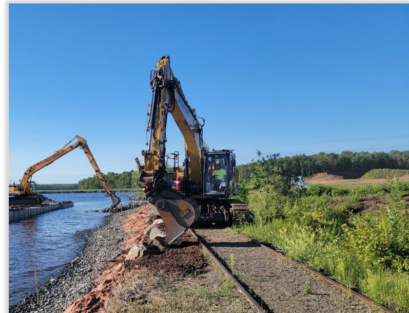
Shoreline protection along with Wire Mill Delta shoreline
