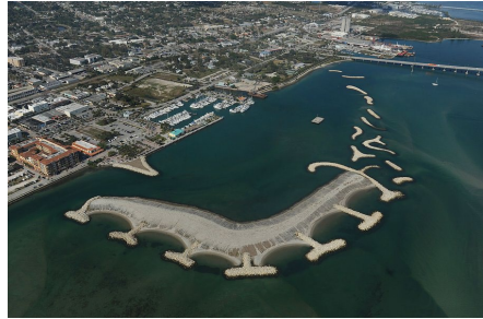
New Island Construction
