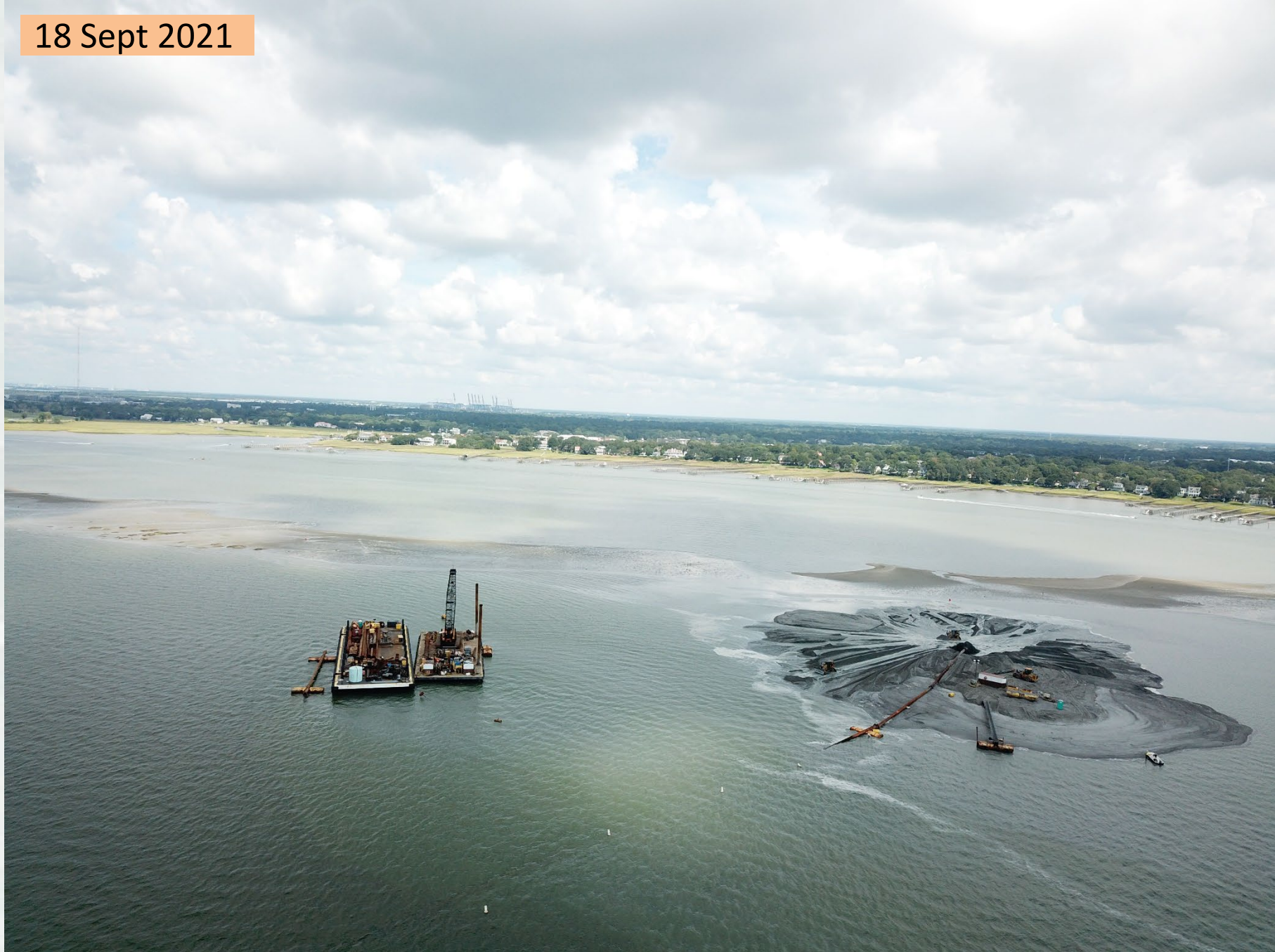
Photo courtesy of Norfolk Dredging Company
