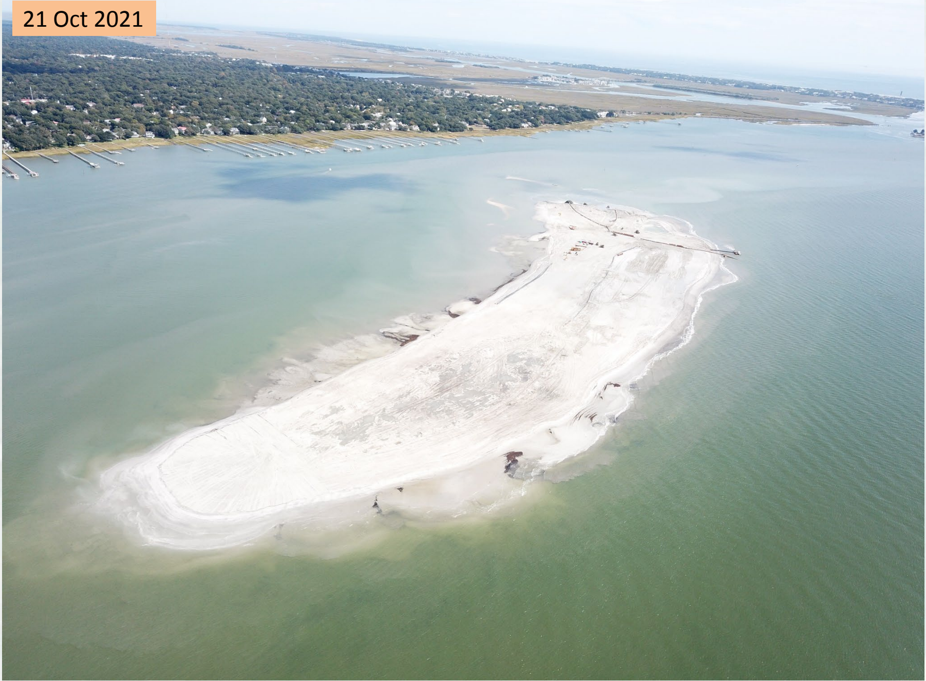
Photo courtesy of Norfolk Dredging Company
