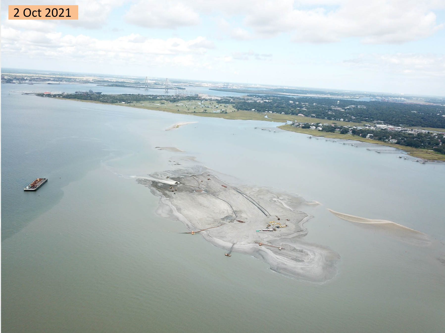
Photo courtesy of Norfolk Dredging Company
