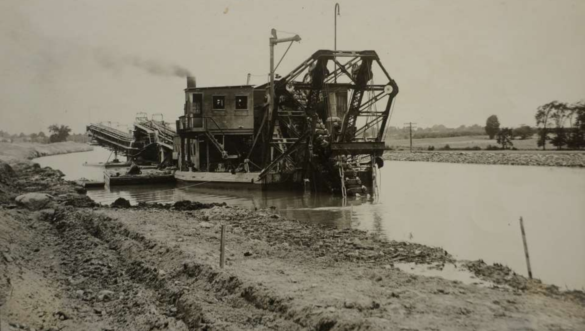
Neg. 7491 Contract 60 Ladder dredge and excavation of prism bend, Sta. 3228+50 Aug. 8-10
