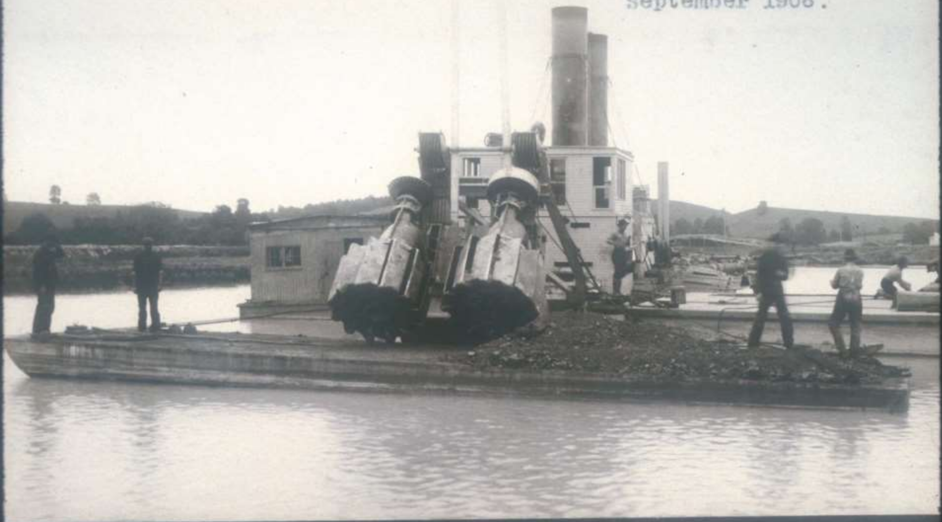
Neg. 1445. View of cutters from under side on Hydraulic Dredge in Operation on Contract No. 5, September 1906.
