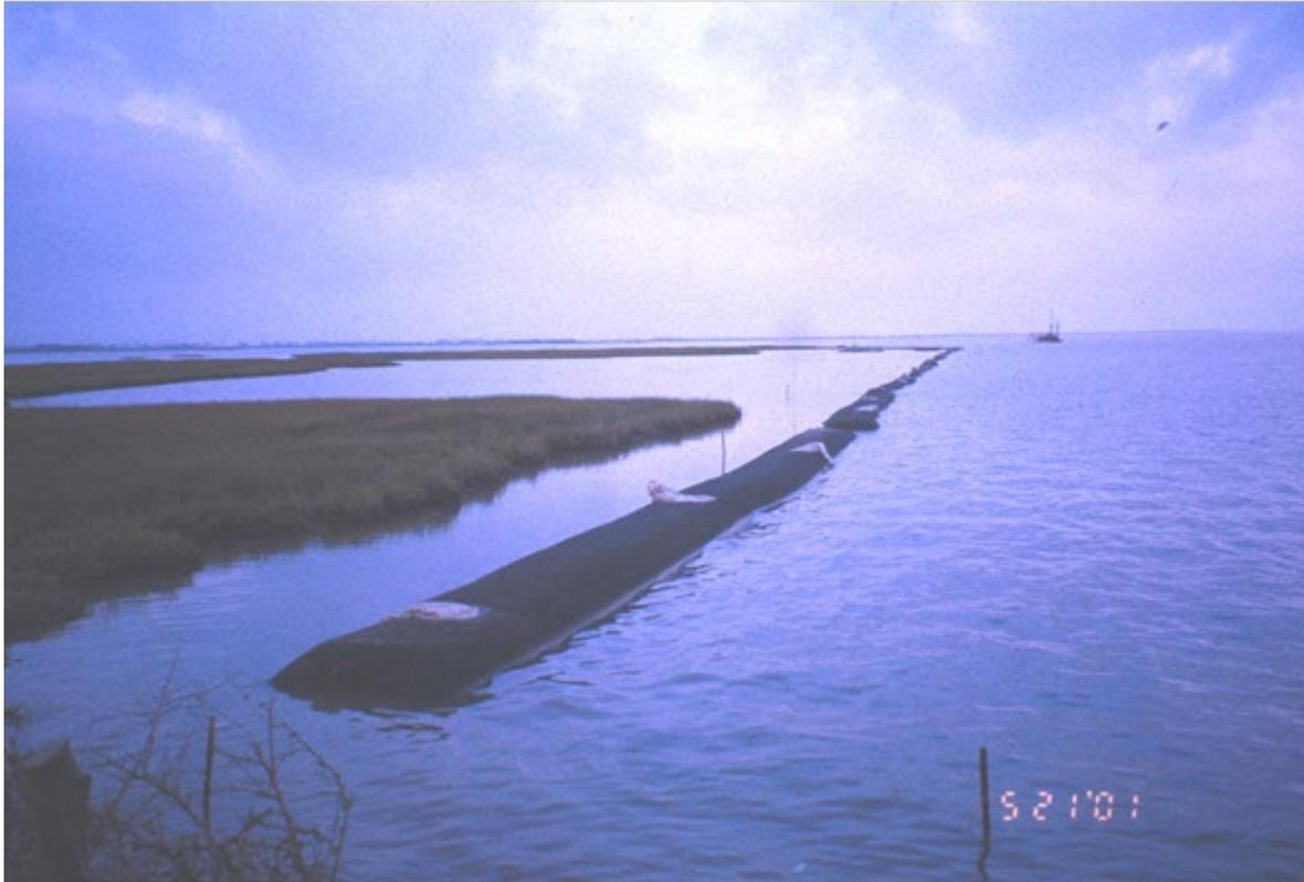
Top: 2,800 linear ft of geotube installed for restored marsh protection. Left: marsh mounds before and after being vegetated with *S. alterniflora*. Photo credit: Cherie O'Brian
