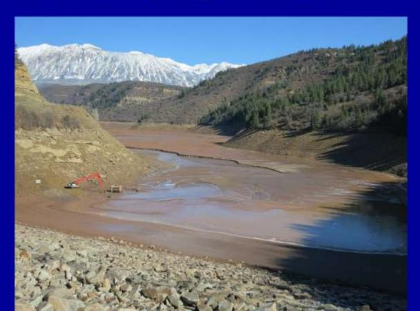
The nation's 90,000 dams and reservoirs constitute a critical component of the country's infrastructure ensuring the stability of water and energy supplies and flood risk management. However, the reservoir storage capacity, essential to meeting these purposes, has been filling with sediment (clay, silt, sand, gravel, and cobble).
