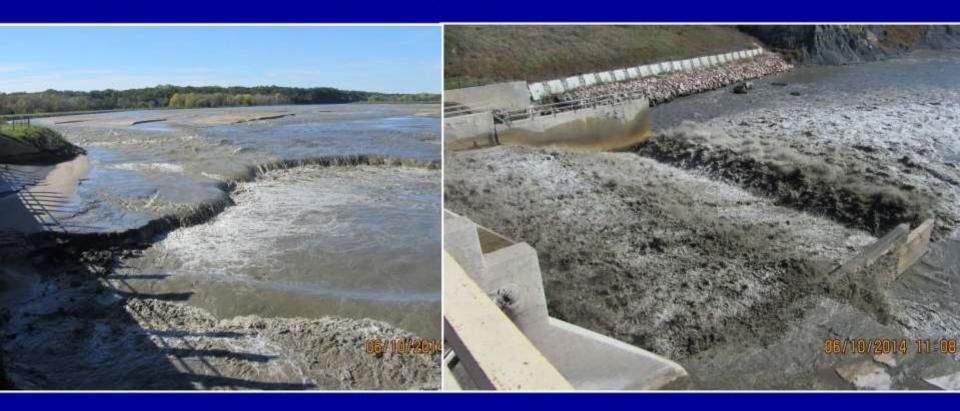
Headcut Erosion in Spenser Reservoir
