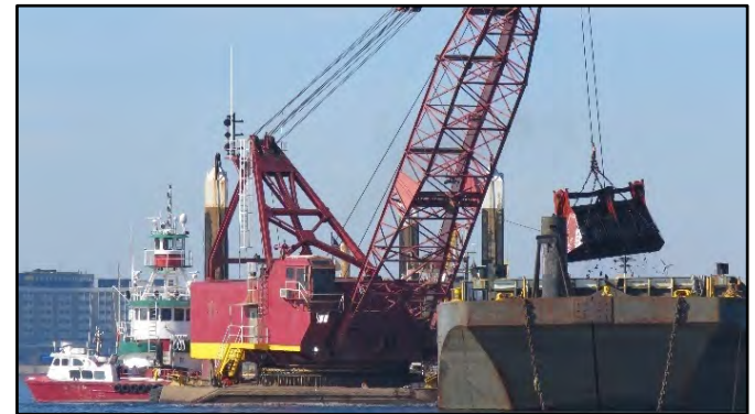
Maintenance Dredging in Ferry Bar Channel (2017)
