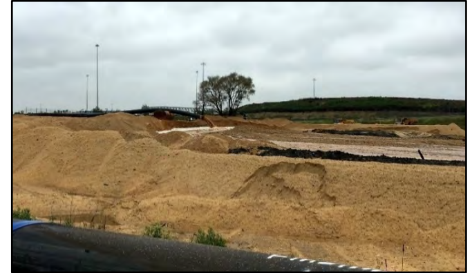
Inflow at Masonville DMCF (2016)
