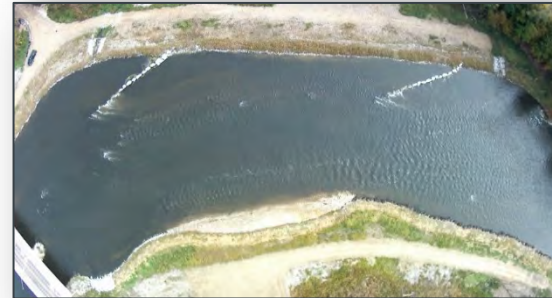
Aerial view after J-hook Installation
