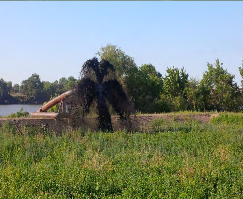
Pump out of Dredge Material into Facility
