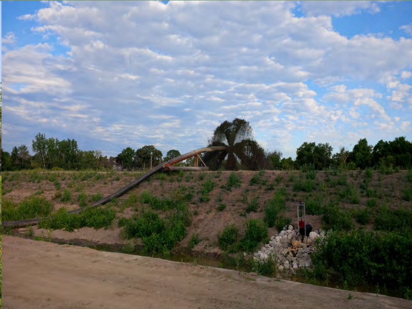
Pump out of Dredge Material into Facility
