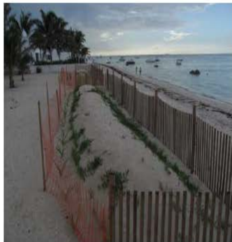
Native plant species placement, sand fence installation and application of the PPB SandFirst for dune stabilization
