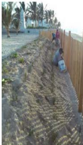
Native plant species placement, sand fence installation and application of the PPB SandFirst for dune stabilization
