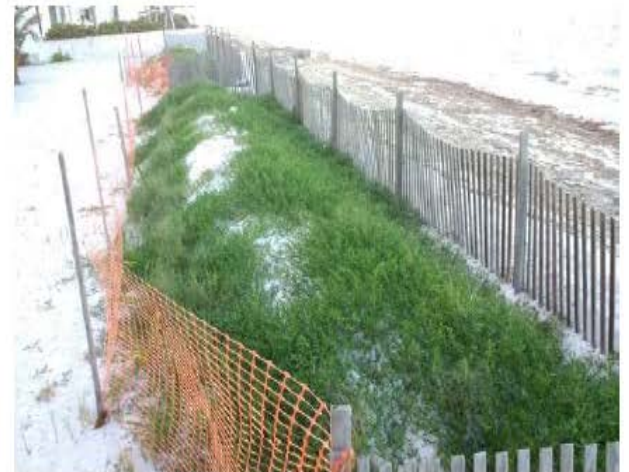
Native plant species placement, sand fence installation and application of the PPB SandFirst for dune stabilization
