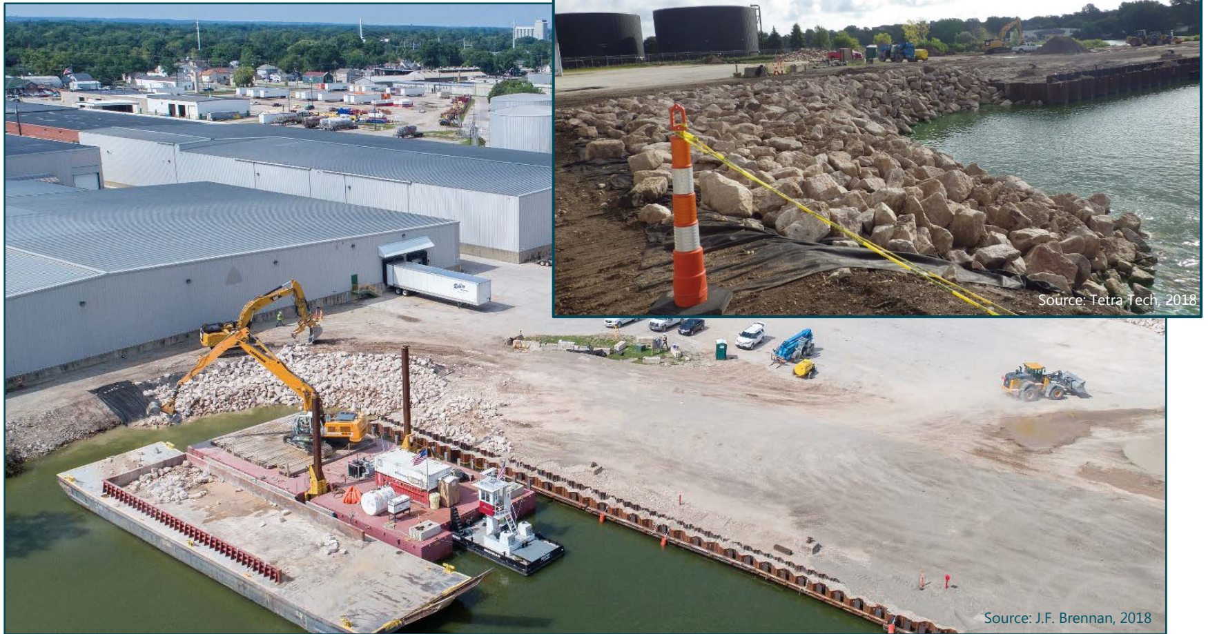
Installation of clean post-dredge buttress
