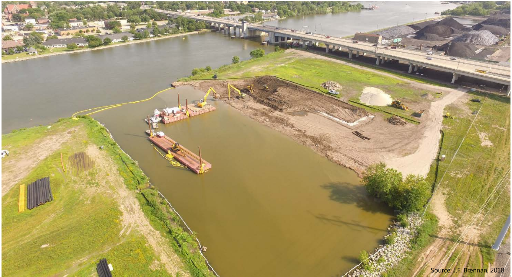
Excavation behind sheetpile walls
