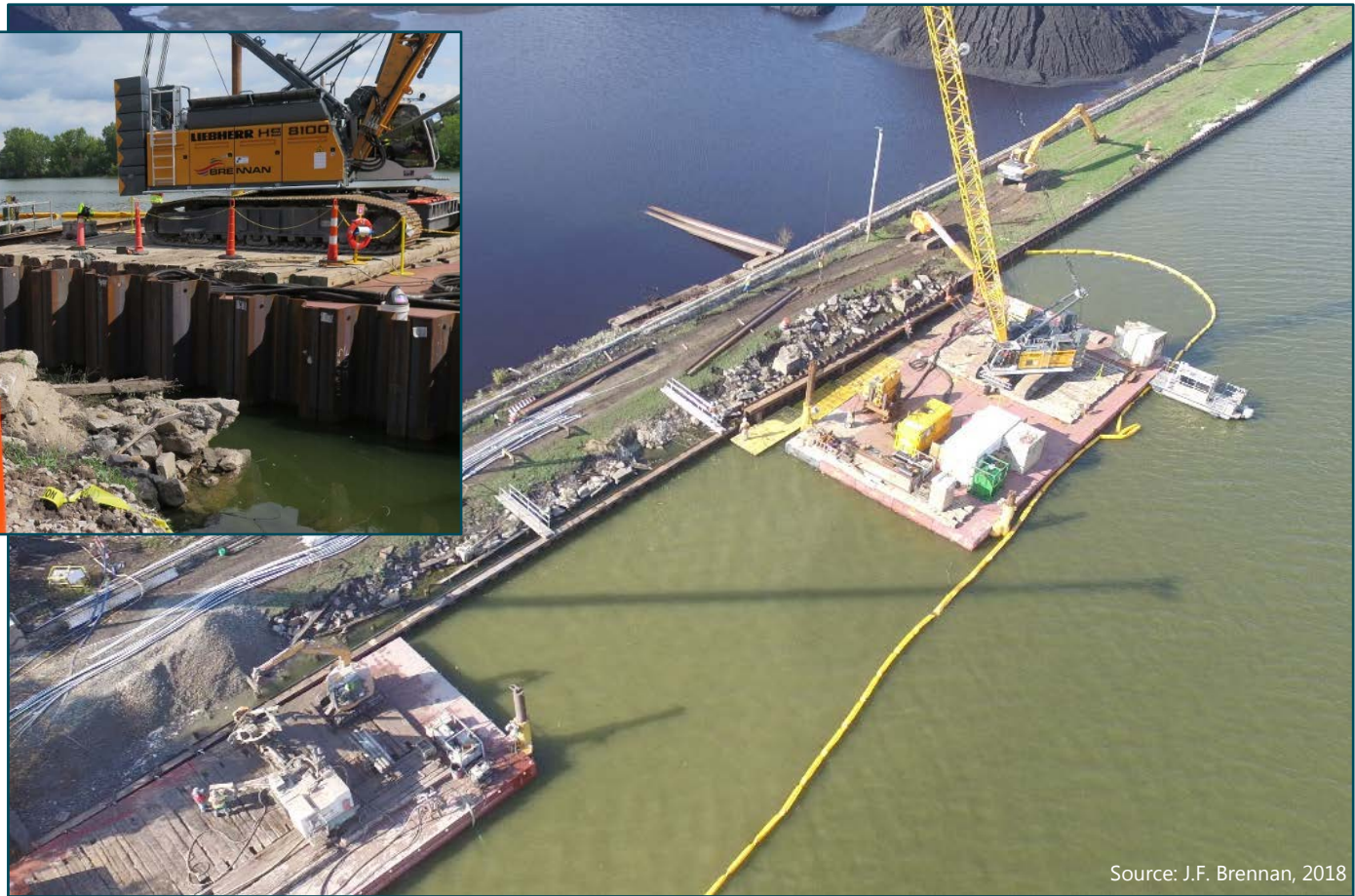
Installation of structural members
