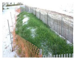
Native plant species placement, sand fence installation and application of the PPB SandFirst for dune stabilization
