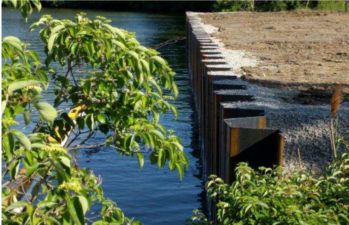
2016 Sheet Pile Installation
