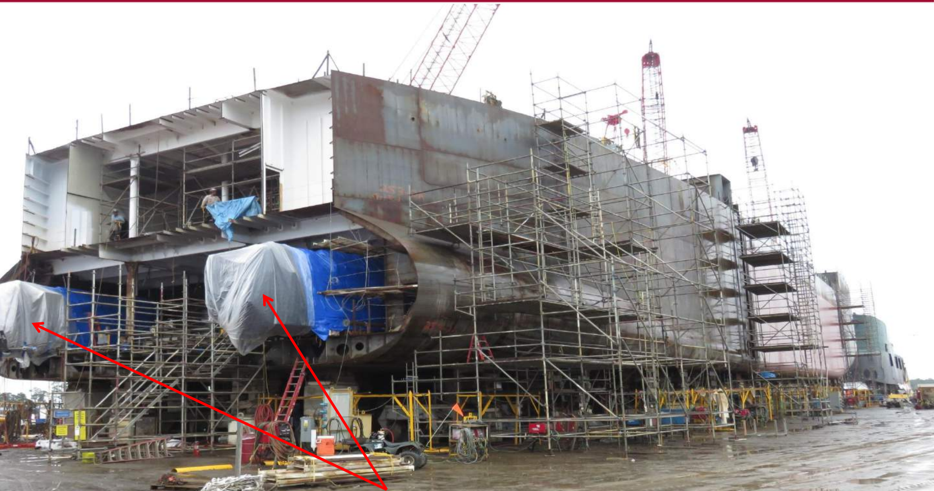
Dredge Pump Engines
