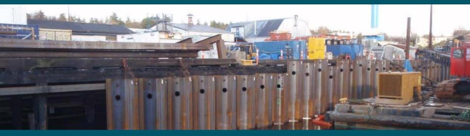
Sheetpile wall prevents resuspension and transport of contaminated under-jetty sediment into Phase 1B area
