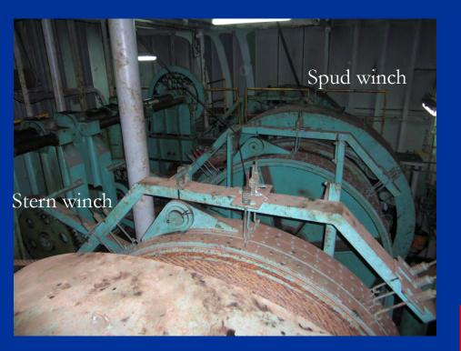
Equipment: Ladder winch Swing winch Spud winch Stern winch Bearing : Electric motor (gear) Reducer Pinion Winch drum Vibration : 15points AE : 33points
