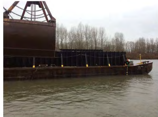
Measuring freeboard of sand barge at sand placement operation.
