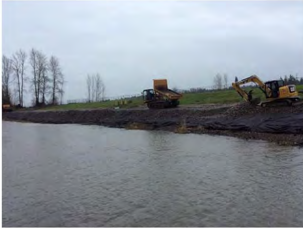
Placing fish mix on shoreline.
