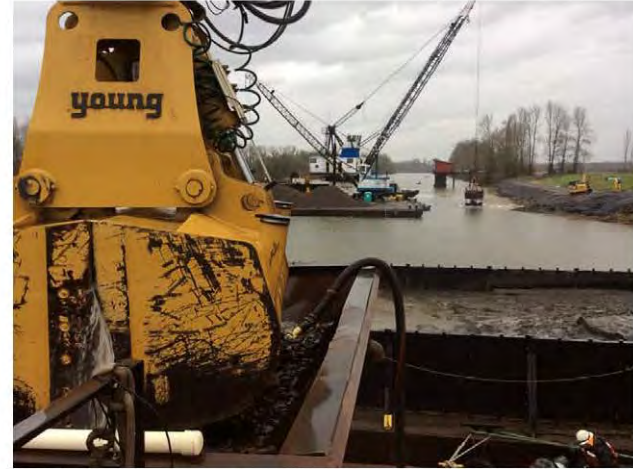
Dredging, sand placement, and fish mix placement during Ecology visit.
