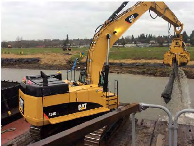
Removing log while dredging.
